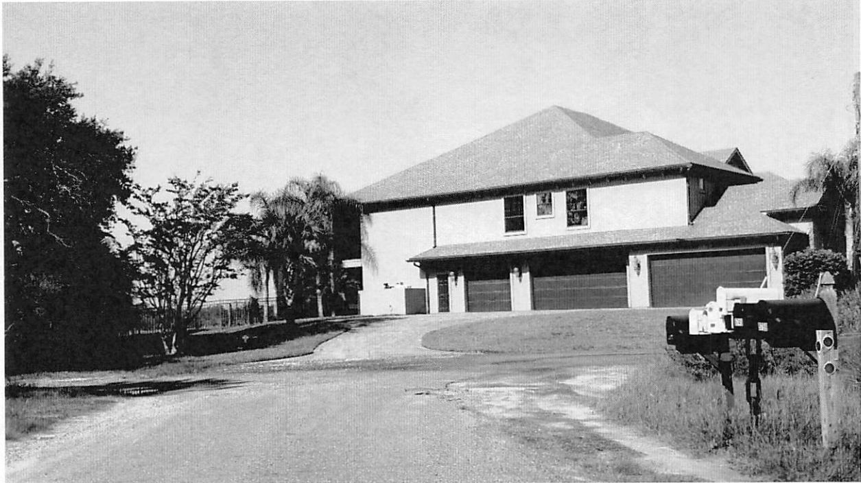
Adjoining property to the north, across Sheffield Road Source: Staff, Planning and Development Department Date: 07.05.17
